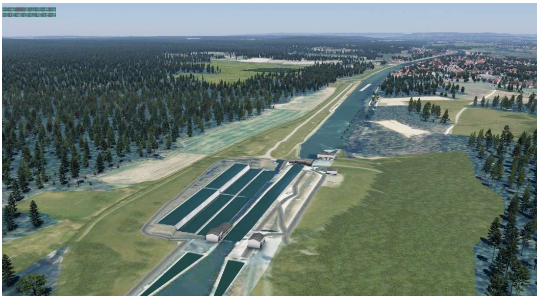
sluices and water bassins
